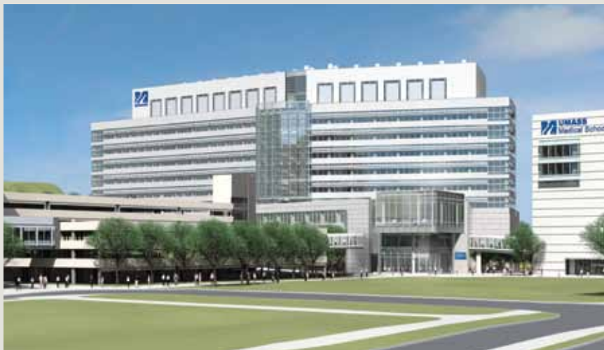
While building the Albert Sherman Center, a new 516,000 sq.ft. research and education facility at The University of Massachusetts Medical School's Worcester campus, the team developed a plan to leverage BIM data for facilities operation and maintenance.
